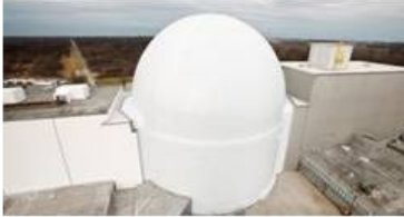
NASA One-of-a-Kind Vibro-Acoustic Research Facility DesignBuild
